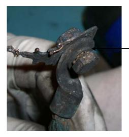
Washer placed under bolt head. No spacer between lug and fuse blade. While examining the various terminations, several of the fused connections were found to be loose (Figure 17).
