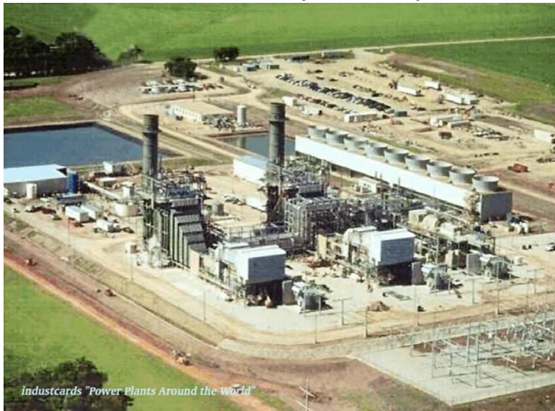
Figure 16. Representative Combined Cycle: McClain Plant (Oklahoma)
