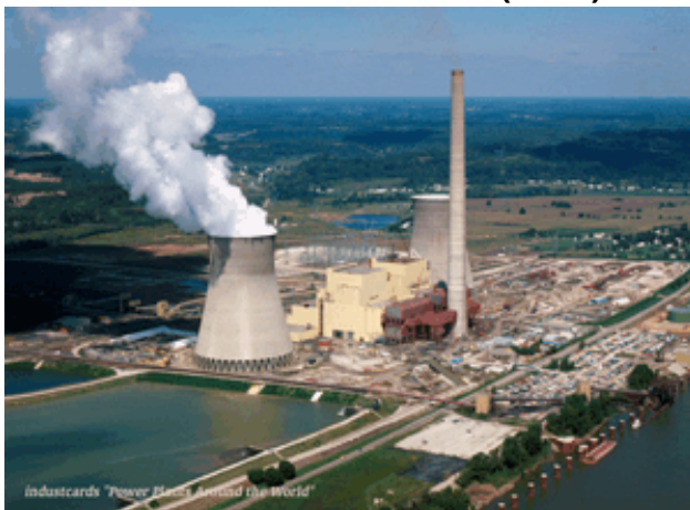
Figure 11. Representative Pulverized Coal Plant: Gavin Plant (Ohio)
