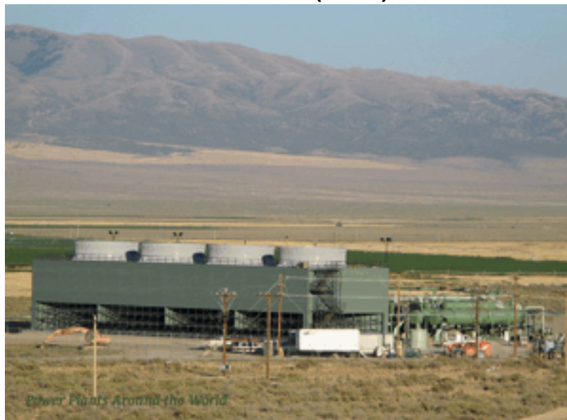
Figure 24. Representative Geothermal Plant: Raft River Plant (Idaho)
